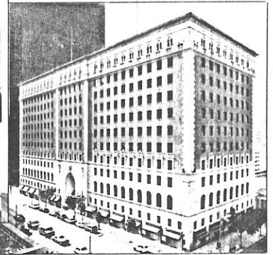
The restored Barker Bros. Building at 818 W. Seventh St. won a Rose for renovation
